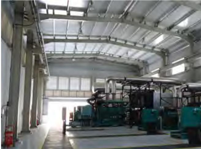
This project is considered one of the huge projects by RAEC this year. The project included exporting, assembling and operating 6 diesel units with total capacity of 7000 kilo Watt. Supporting parts and distribution boards were also provided .In addition the same project comprised constructing two fuel tanks with a capacity of 500 m3 each.
